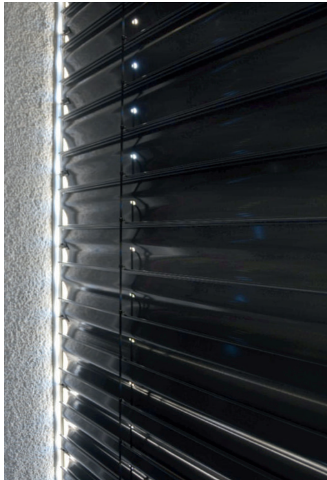
Figure 6: Permissible entry of scattered light through the lateral guide
